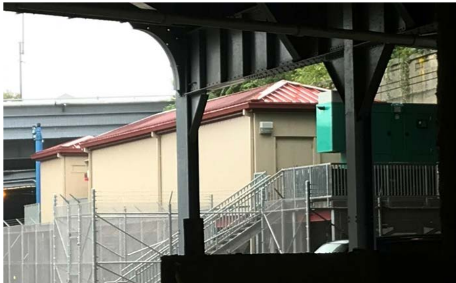
Raised SIR Signal House, St. George
