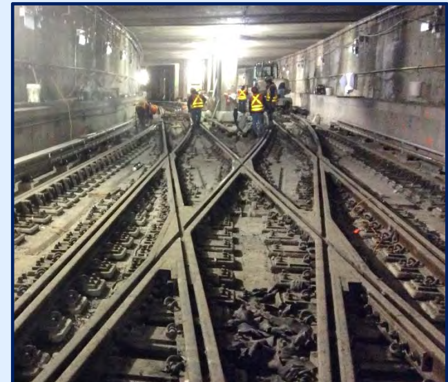
Installing diamond crossover
