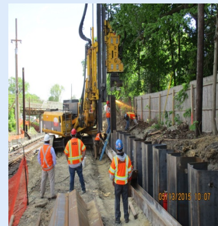
Building Retaining Walls for Great Neck Pocket Track
