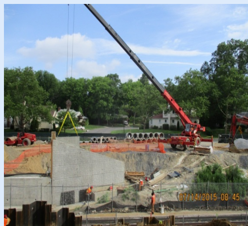
Building Retaining Walls for Great Neck Pocket Track
