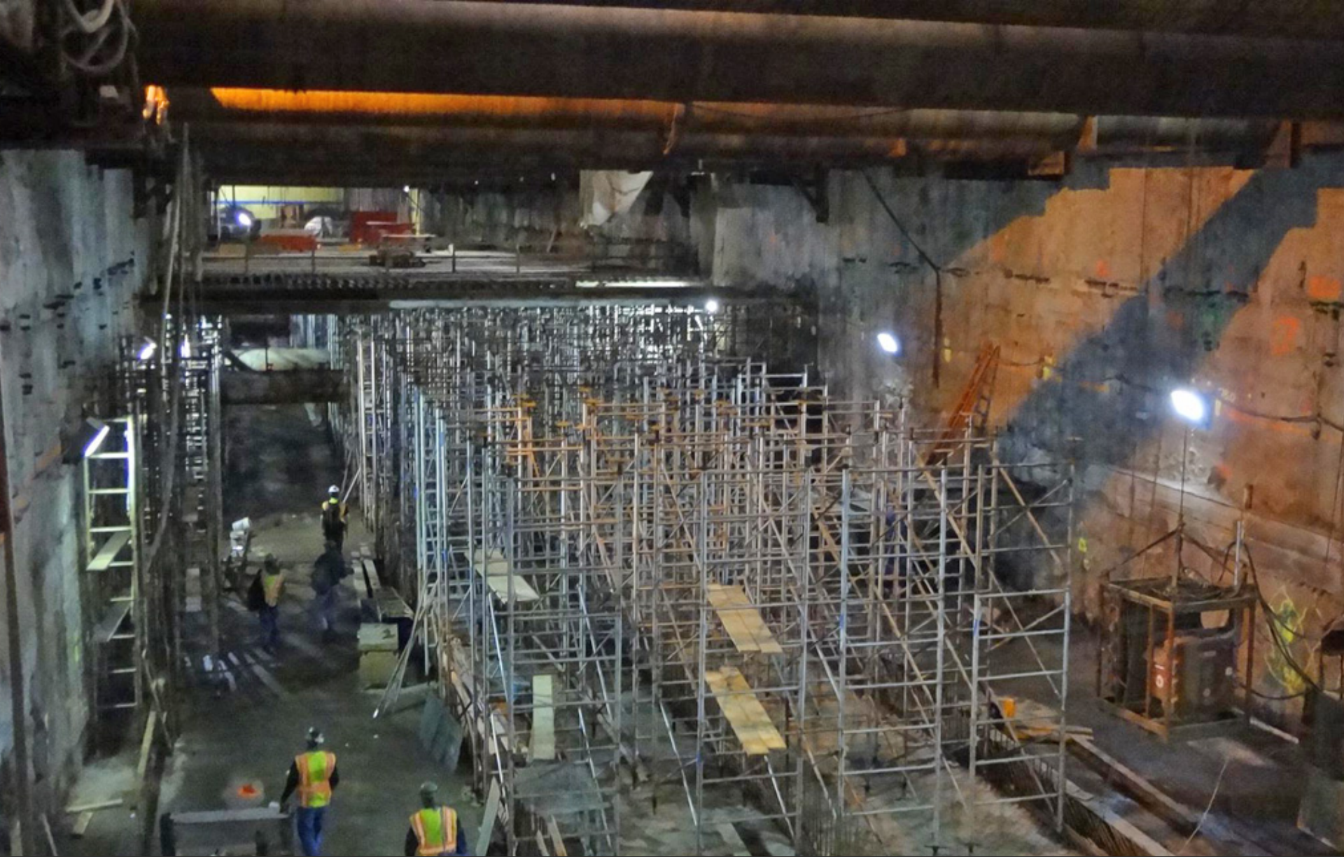
Mezzanine slab shoring tower – April 2013
