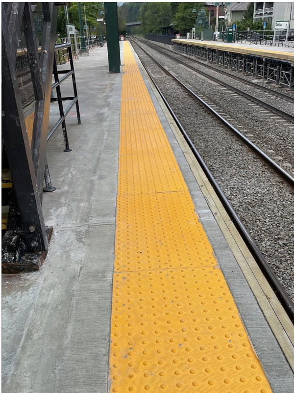
Platform upgrades at Garrison Station
