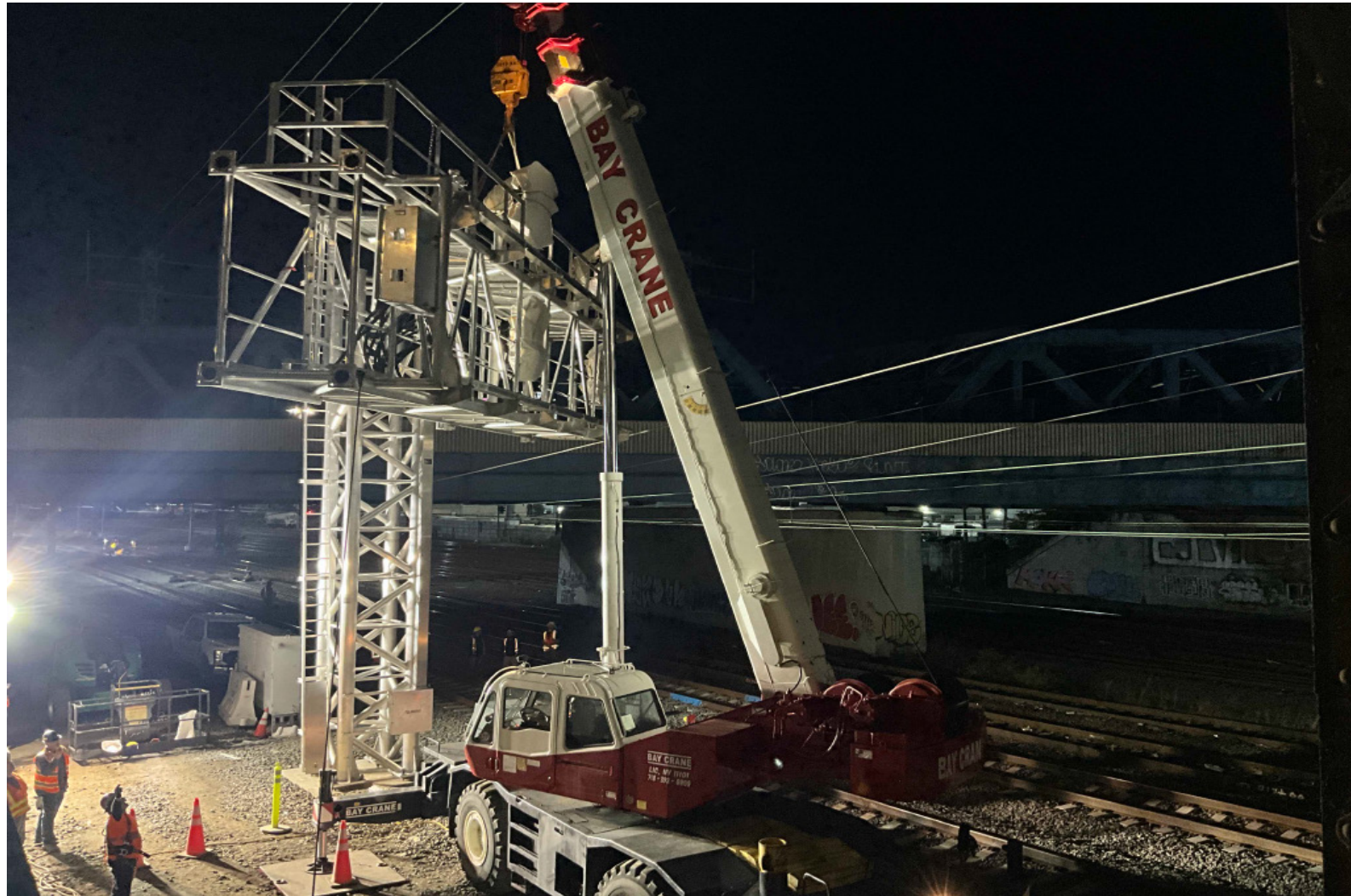
Above: New signal bridge at Leggett Interlocking - December 2024
