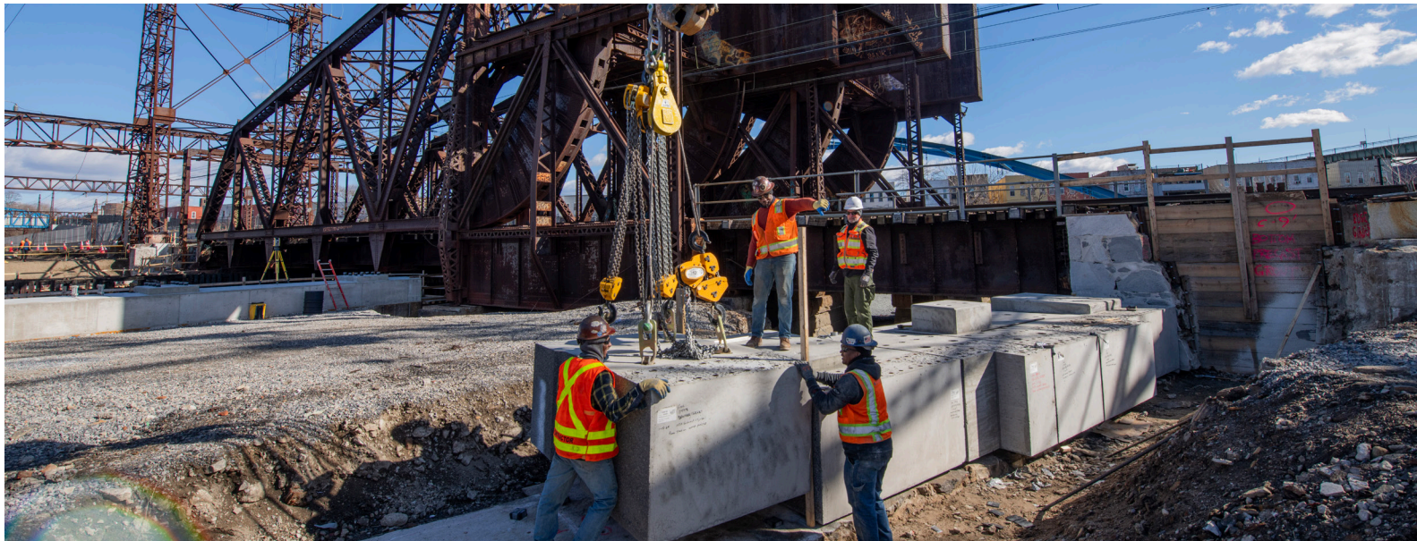
Crews receive the pre-cast concrete for Bronx River Bridge, February 2025
