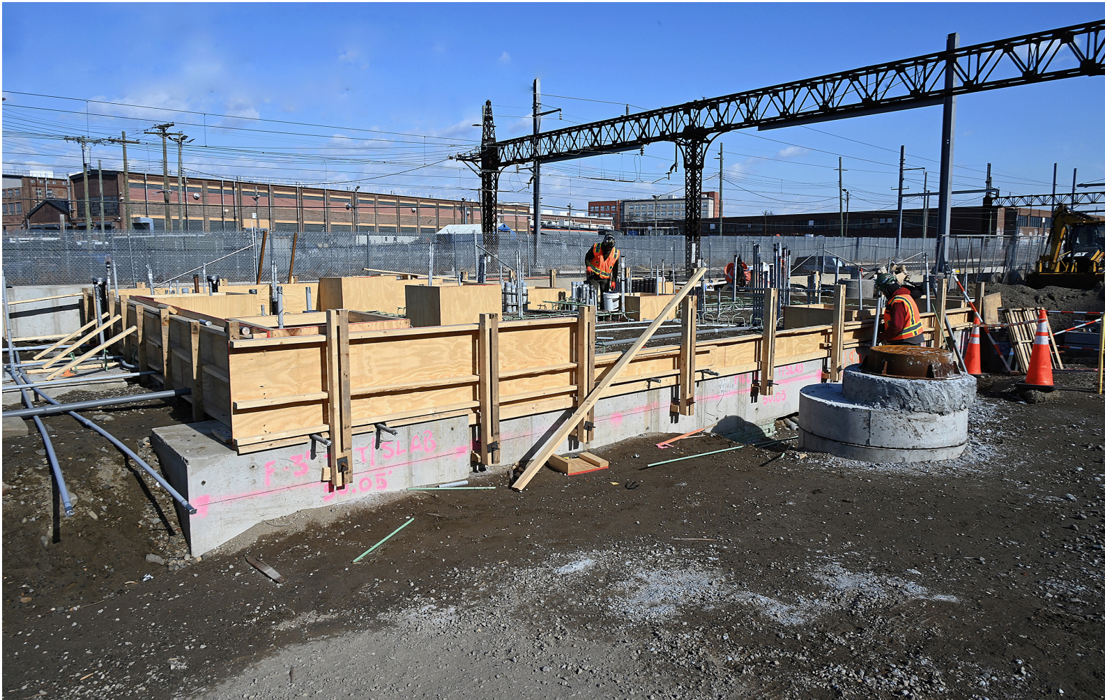
Crews working at the Parkchester / Van Nest Station Site - January 2025
