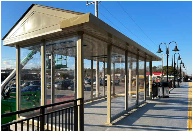
Station improvements to Mastic-Shirley are almost complete
