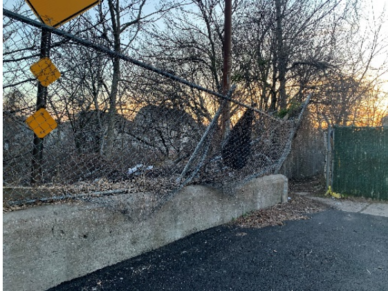
View south of open-cut portion of the proposed alignment from the dead-end at Erastina Place
