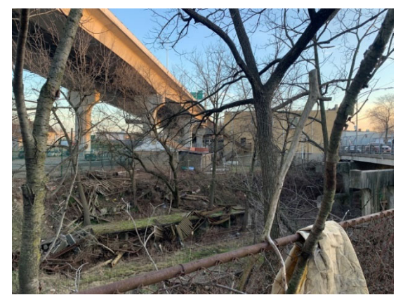
View north of the proposed alignment situated in the open-cut along Eaton Place
