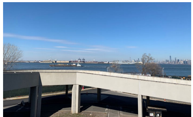
View north of existing ramp from Richmond Terrace to the garage at the former New York Wheel site
