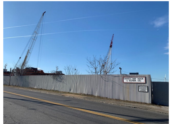
View west of the Caddell Dry Dock property from Richmond Terrace; proposed alignment obstructed by existing fencing
