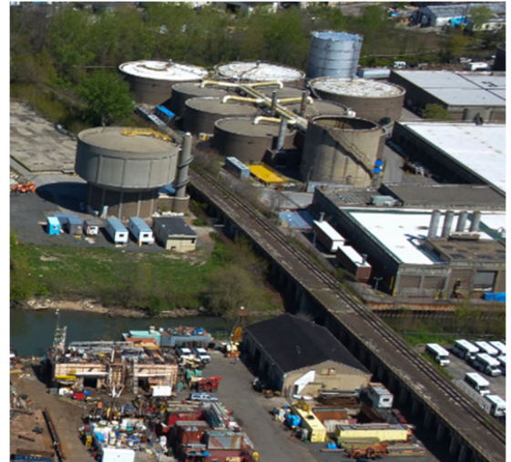
Viaduct and Port Richmond Wastewater Resource Recovery Facility
