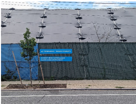
View along Richmond Terrace and chain-link fencing at the site of the Atlantic Salt Terminal
