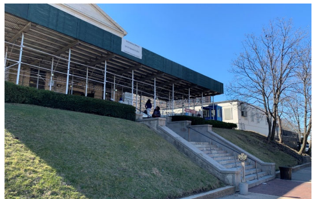
View northwest of the Staten Island Family Courthouse
