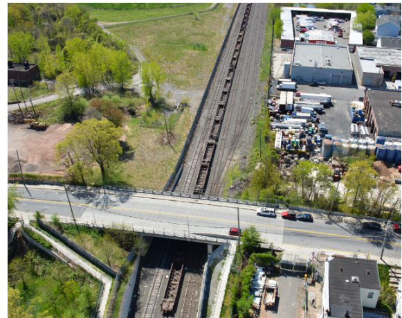
South Avenue Bridge, existing pedestrian walkway and proposed Arlington Station site at left
