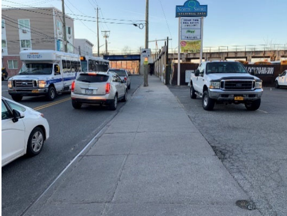
View north of the viaduct along Richmond Terrace
