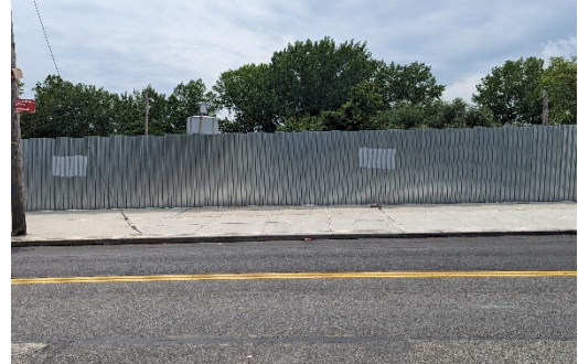
View west from South Avenue from just south of the bridge over the existing right-of-way
