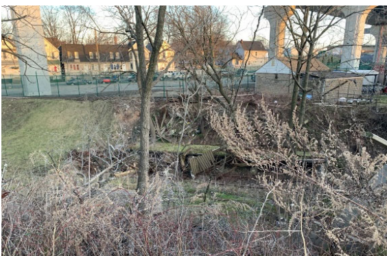
View southeast of vegetative growth and garbage within the open-cut portion of the proposed alignment
