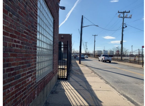
View of brick Con Ed facility facing west along Richmond Terrace
