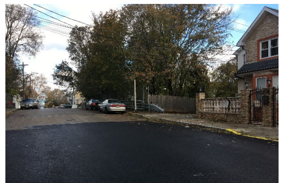
View north of open-cut portion of the proposed alignment from Simonson Avenue and roadway bridge
