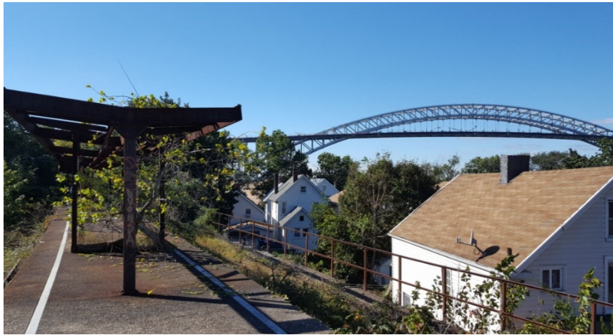
Viaduct: View of remnant station on viaduct section of ROW
