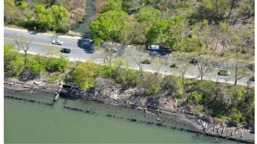
At-Grade: View of ROW and destabilized shoreline near Snug Harbor
