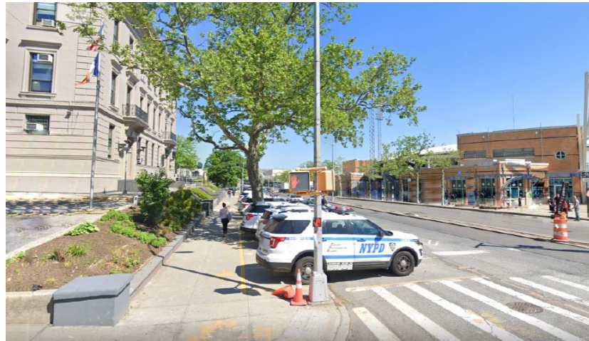
No-Action Condition 120th Police Precinct view from Wall Street
