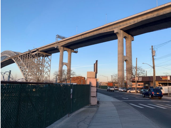
View northeast of the Bayonne Bridge from Richmond Terrace
