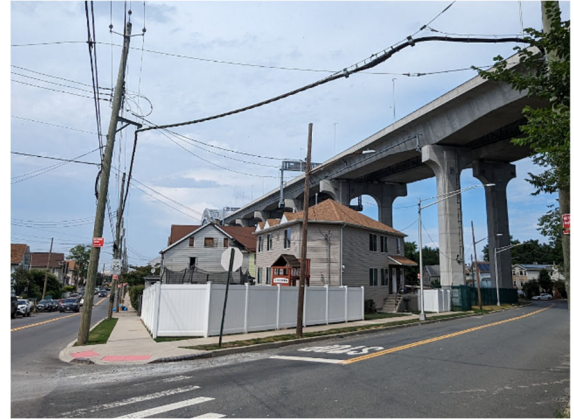
View north of the Bayonne Bridge approach from the intersection of Morningstar Road and Newark Avenue
