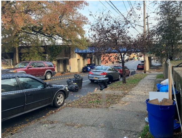
View northeast of the viaduct along Park Avenue
