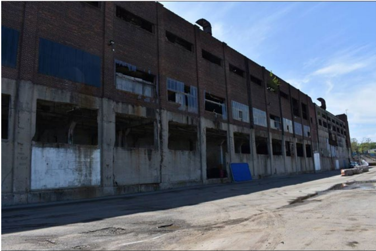
Figure 9.7.1 North face of multi-story building atop the tunnel structure (pre-demolition)
