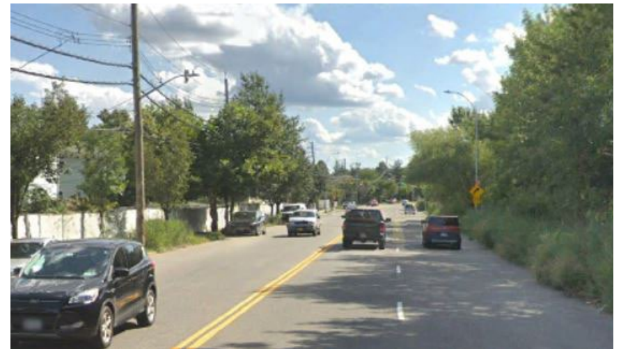
On-Street Mixed-Traffic: View of South Avenue
