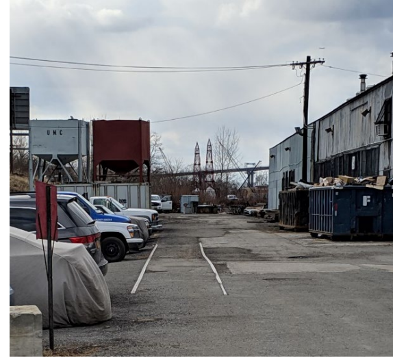
View of remnant track & ROW through Caddell Dry Dock & Repair
