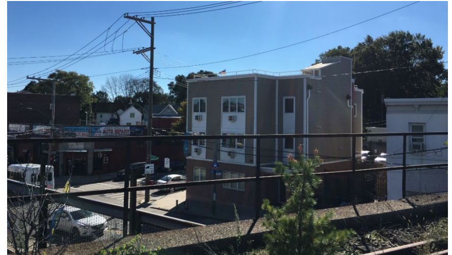
Viaduct: View of Richmond Terrace looking south from viaduct
