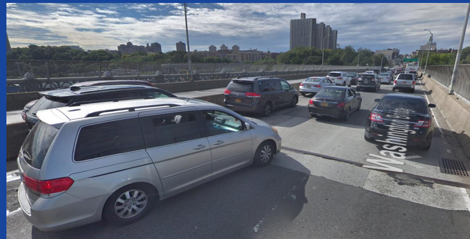
Washington Bridge, Looking East
