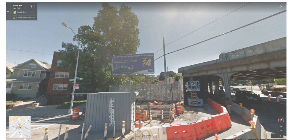
1 NORTH SIDE OF TRACKS LOOKING SOUTH EAST WOODHAVEN BLVD
