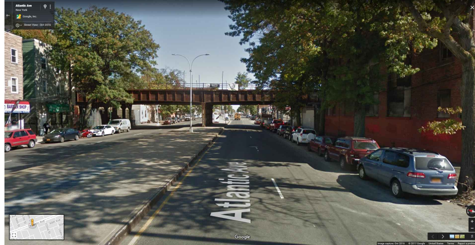
9 WEST SIDE OF TRACKS LOOKING EAST ATLANTIC AVE
