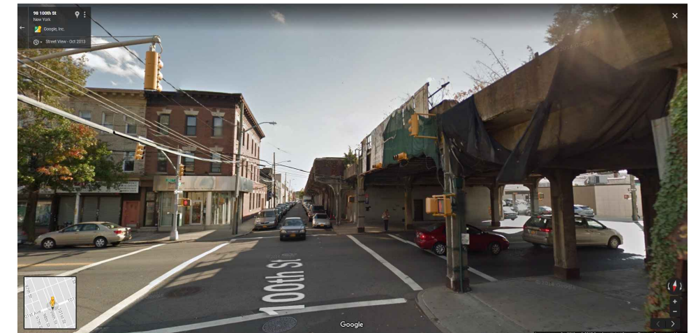
6 EAST SIDE OF TRACKS LOOKING SOUTH EAST 100TH STREET AVENUE AND 101ST AVENUE
