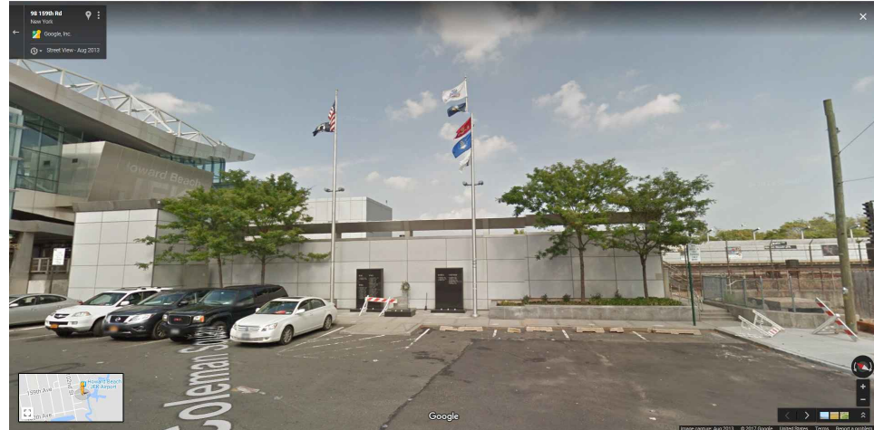
5 WEST SIDE OF TRACKS LOOKING EAST 159TH RD
