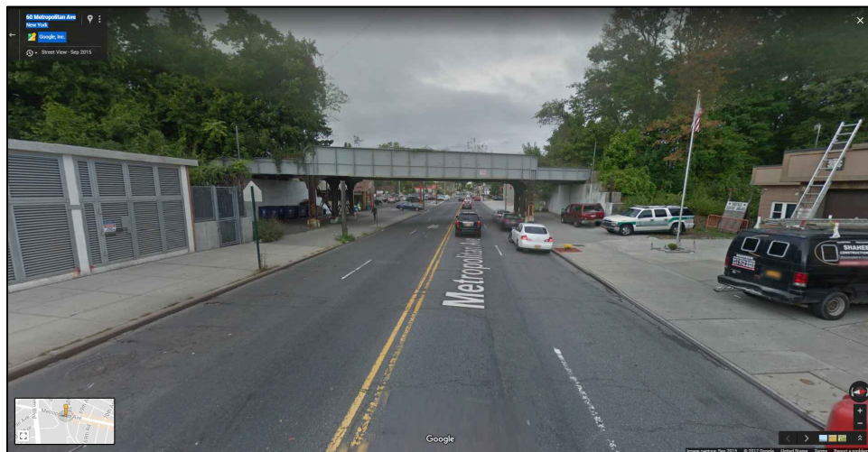
2 EAST SIDE OF TRACKS LOOKING SOUTH WEST METROPOLITAN AVE
