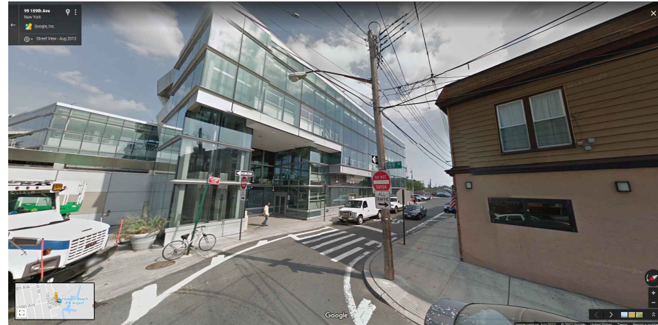
4 WEST SIDE OF TRACKS LOOKING SOUTH EAST 159TH AVE
