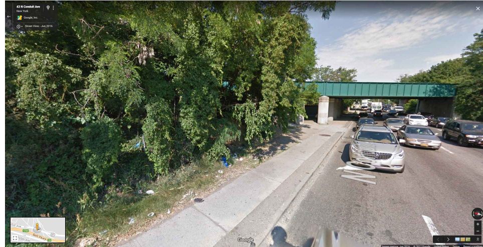
5 WEST SIDE OF TRACKS LOOKING NORTH EAST N CONDUIT AVE
