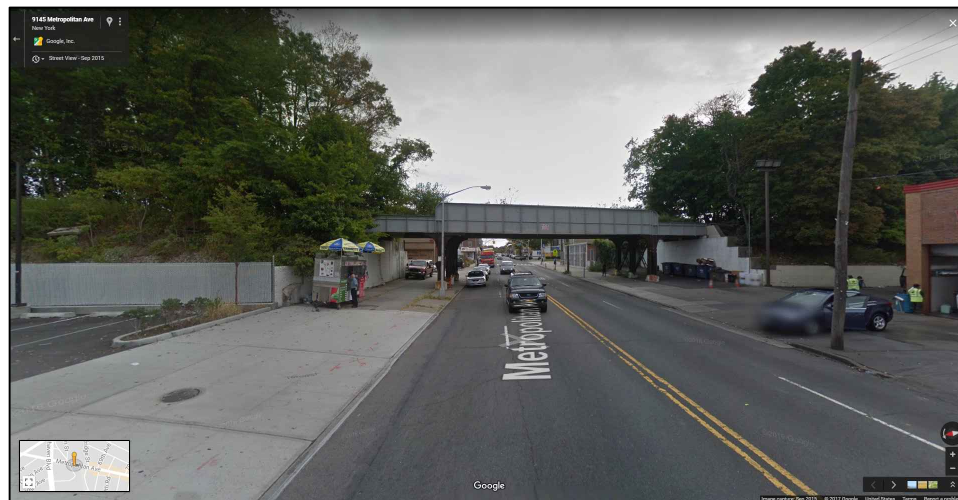
4 WEST SIDE OF TRACKS LOOKING EAST METROPOLITAN AVE
