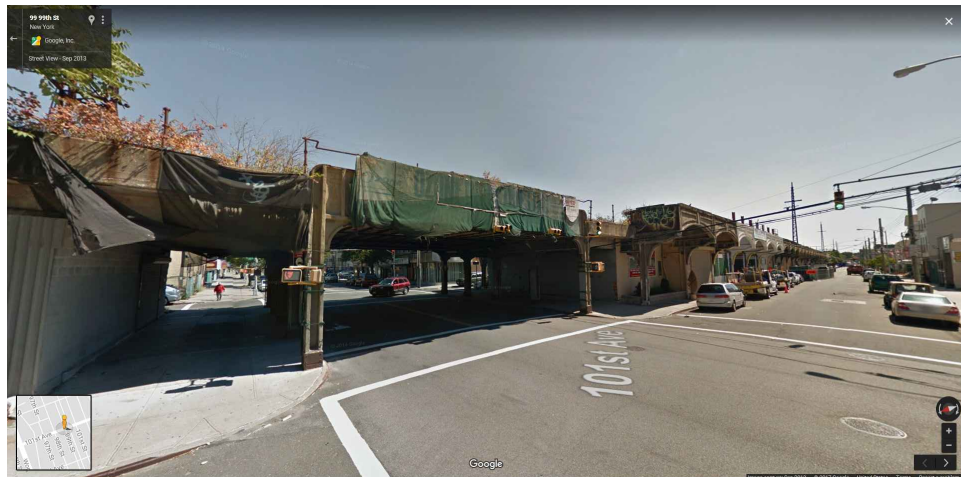
2 WEST SIDE OF TRACKS LOOKING SOUTH EAST 101ST AVENUE AND 99TH STREET
