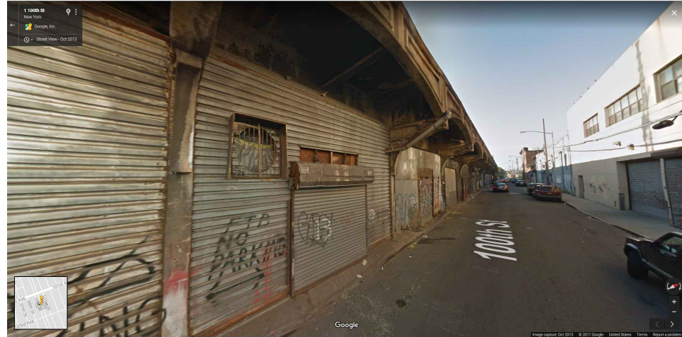
9 EAST SIDE OF TRACKS LOOKING NORTH EAST 100TH STREET
