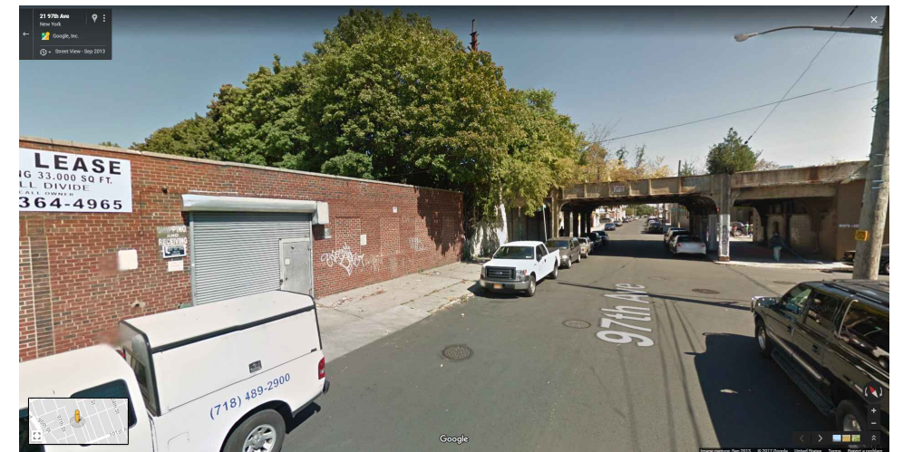
6 WEST SIDE OF TRACKS LOOKING NORTH EAST 97TH AVE
