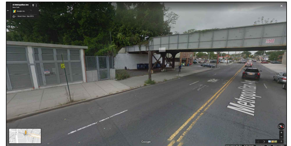
1 EAST SIDE OF TRACKS LOOKING SOUTH WEST METROPOLITAN AVE
