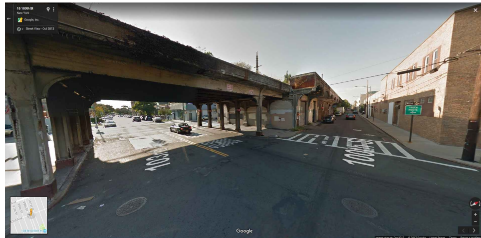
7 EAST SIDE OF TRACKS LOOKING NORTH EAST 100TH STREET AVENUE AND 103RD AVENUE
