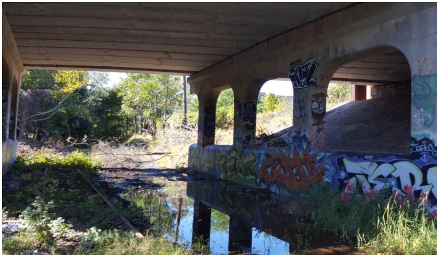
Open-Cut: View of overhead bridge and abutments in open-cut section
