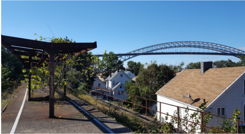
Viaduct: View of remnant station on viaduct segment of ROW
