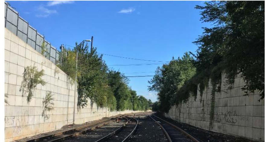
Open-Cut: View of western portion of open-cut section (freight use)
