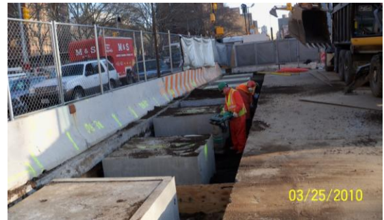
Installation of splice boxes between 96 th and 97 th Streets
