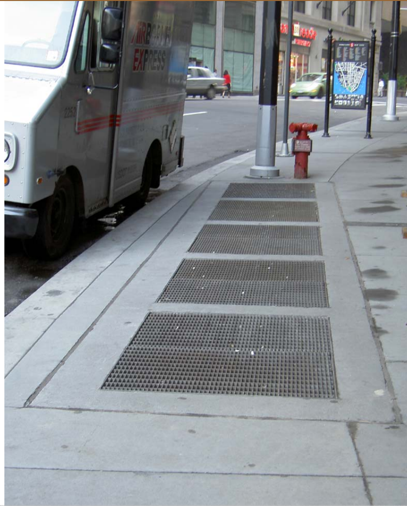
Existing Subway Vent Gratings
